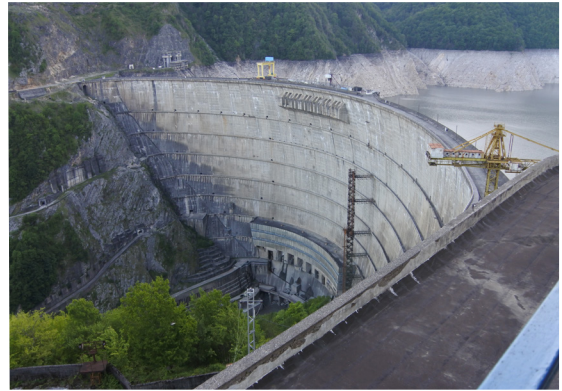
Fig. 1: The 277 m high arch dam of the Enguri dam in Georgia (Image credit: KIT/AGW).
