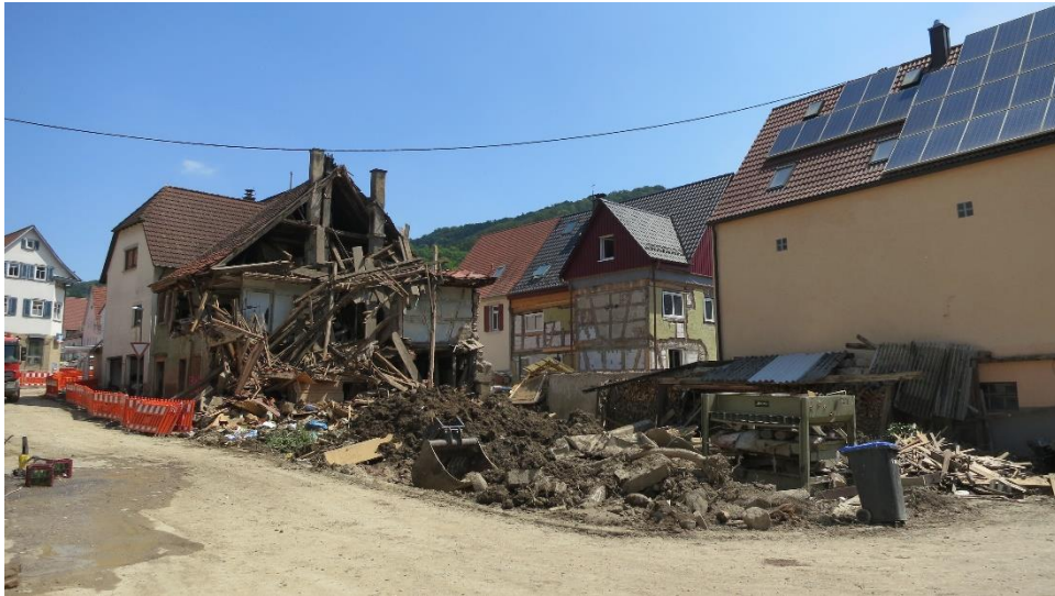
Figure 13: Buildings destroyed by flow attack and debris impact in Braunsbach.
