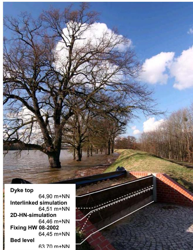
Figure 3: Differences in calculated water levels using the 2D reference model and the interlinked model as well as exemplary analysis of a dyke opening near Wörlitz for the August 2002 flood.
